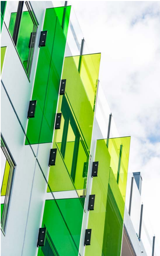
Custom laminated 17.52mm heat strengthened glass panels with Vanceva@coloured interlayers - Baxter St Apartments
